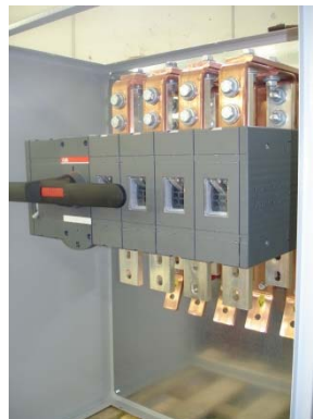
Motorized switches (INTERNAL VIEW)
