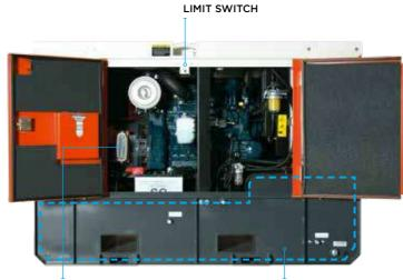
STANDARD BATTERY ISOLATOR & OPTIONAL CHARGER FUEL TANK 24 HOUR RUN TIME (BUNDED 110%)
