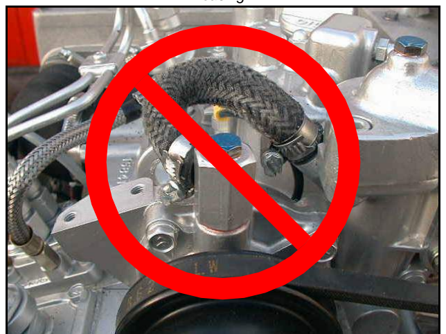
Fig. 7.10-5: Ventilation screw above the cooling water pump casing
