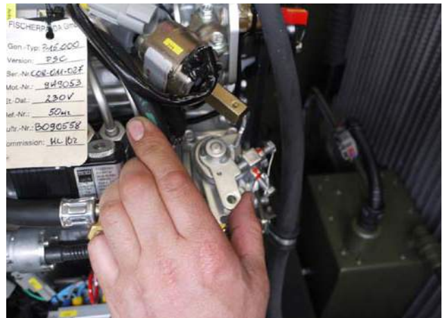
Fig. 7.16-9: Stop solenoid
