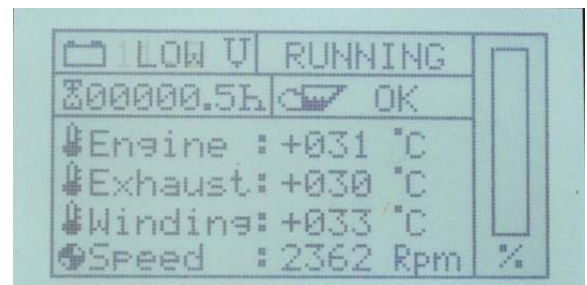
Fig. 14.1.1-1: Warning: „Battery power too low“
