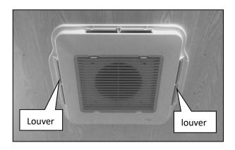
Ajust direction and angle of louver by moving the raised piece in the center of louver. Louvers on opposite sides are symmetrical.
