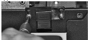
13. Install the new hinge. Fasten with two screws.
