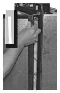
4. Carefully place door on a soft protective material to prevent any damage to the door.
