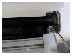
Stainless Steel lugs holding the blind assembly to the window.
