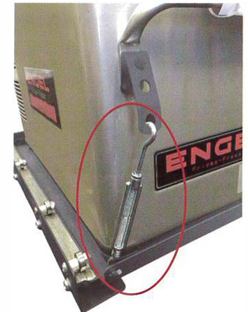
Tie Down Brackets And Turn Buckles Installed
