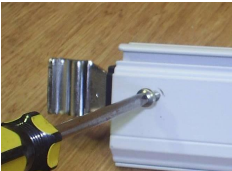
Image 2: Extension Arm Fitting
